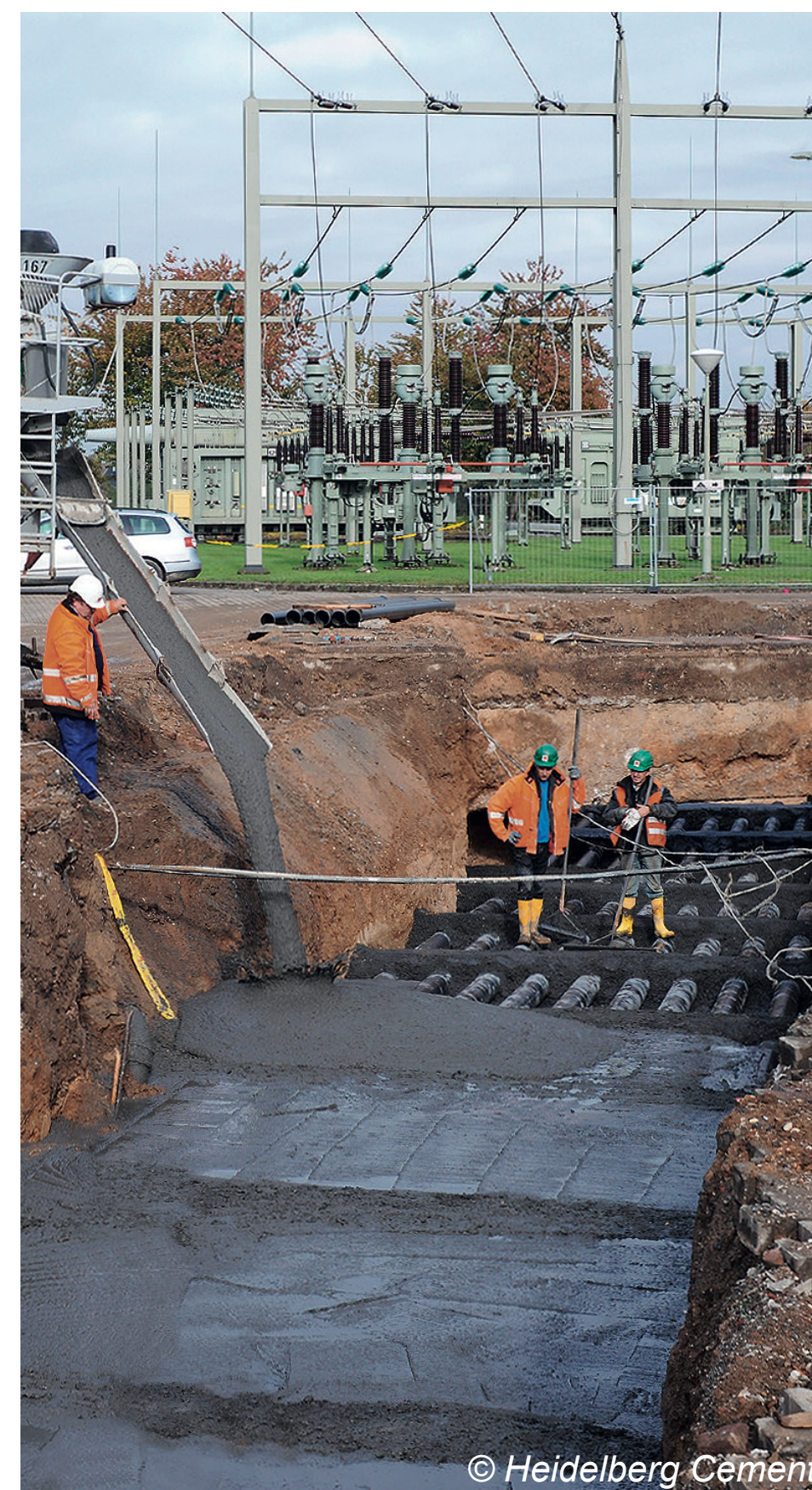
Thermal concrete in underground power line application.
