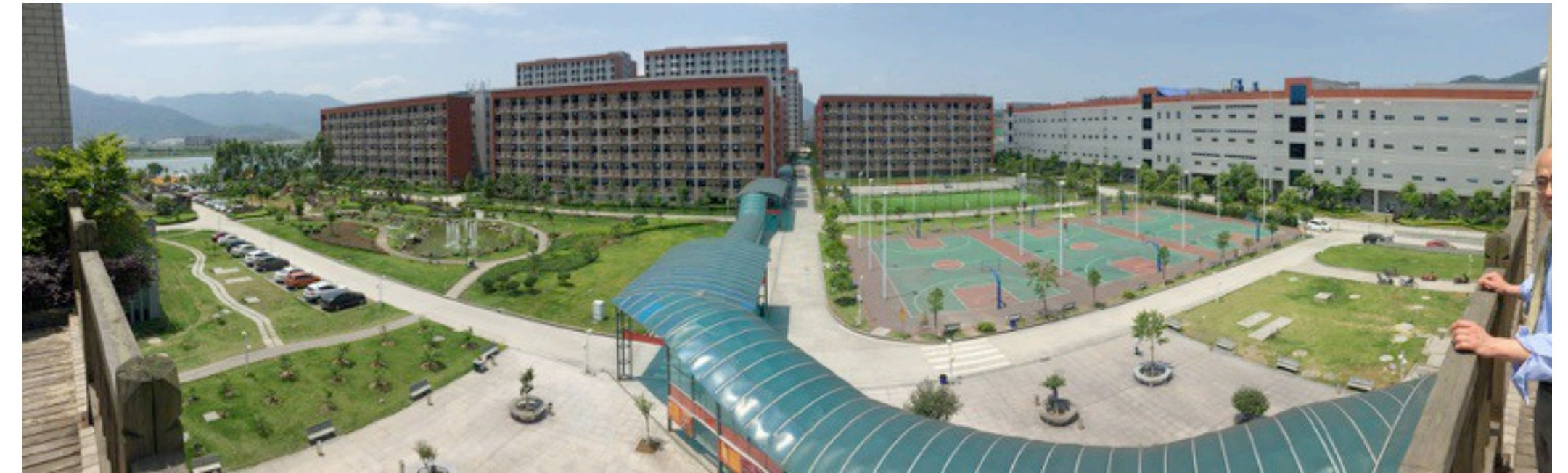
Live-in factory facilities of global leading Li-ion battery manufacturer, China
