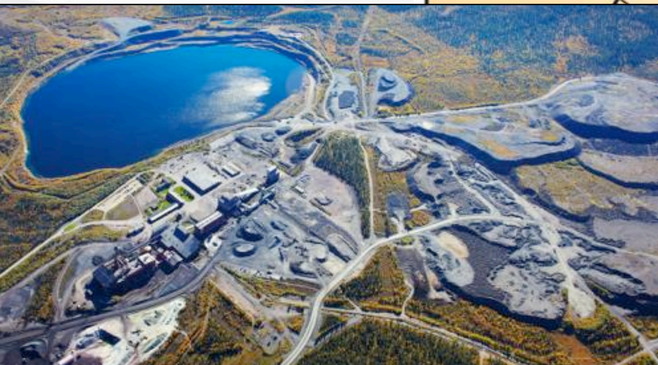
Svappavaara magnetite mine and mill owned by LKAB. Photo©Fredric Alm/LKAB
