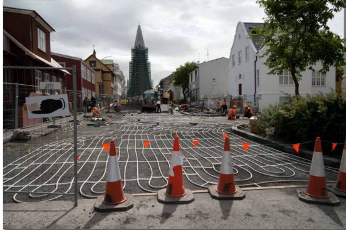
Municipal level road heating installation
