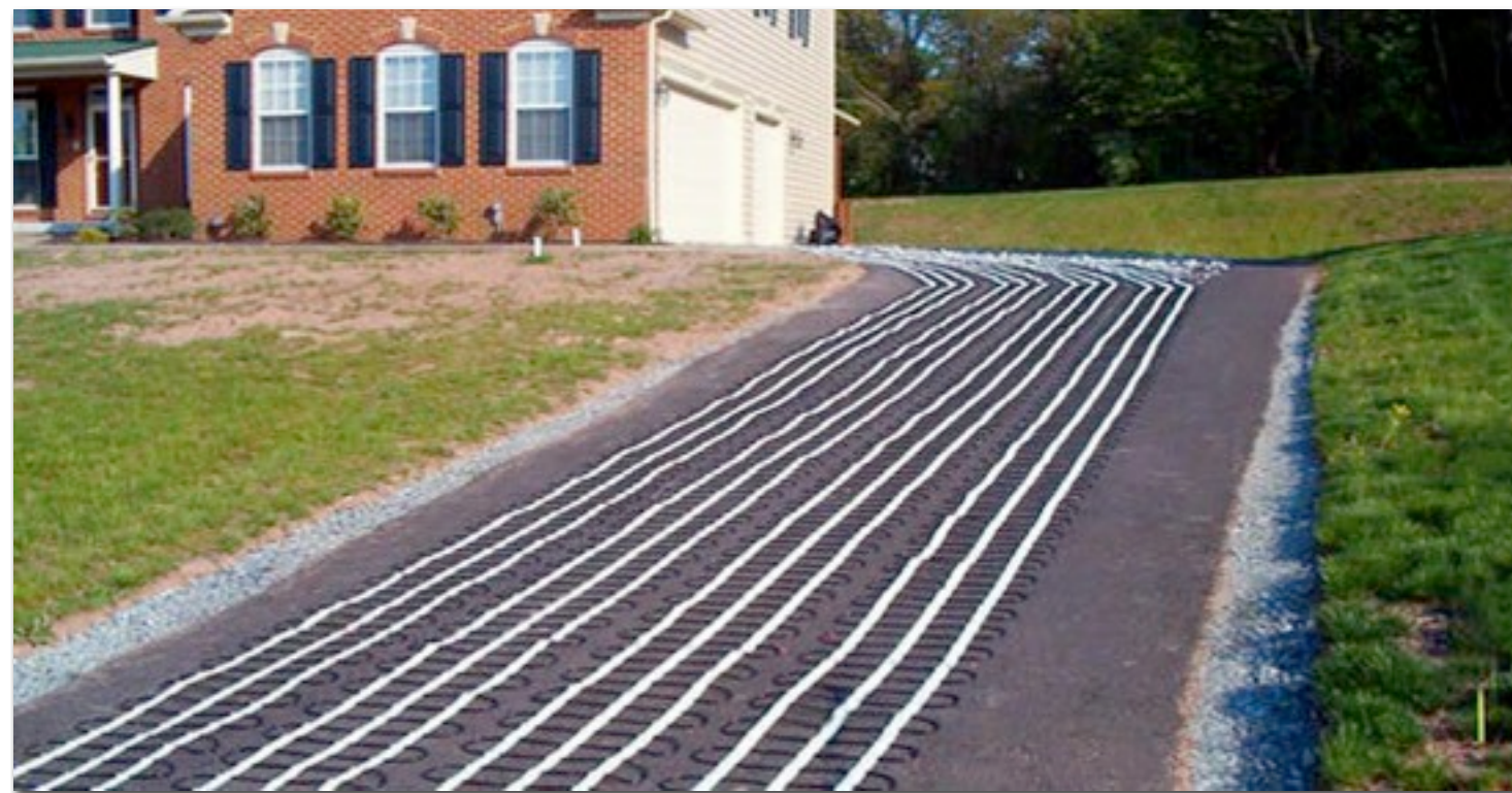
Domestic driveway heating installation
