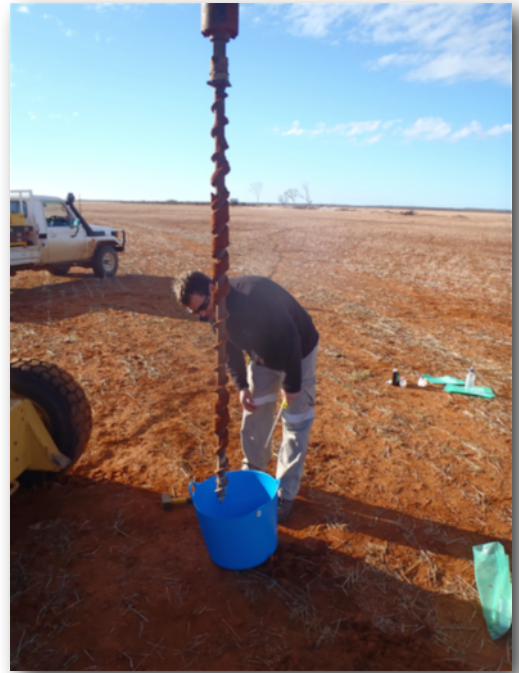
Photo 4. Augering completed as part of the detailed surface geochemical orientation surveys.
