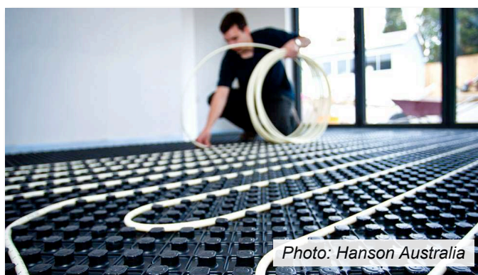
Figure 4 Traditional plumbed underfloor heating - can be replaced by long life solid state conductive concrete.
