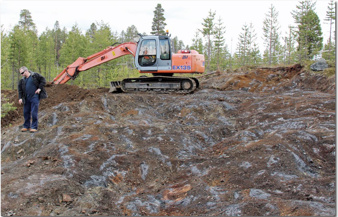
Figure 4 - High grade ore zone exposed after soil clearing/stockpiling.
