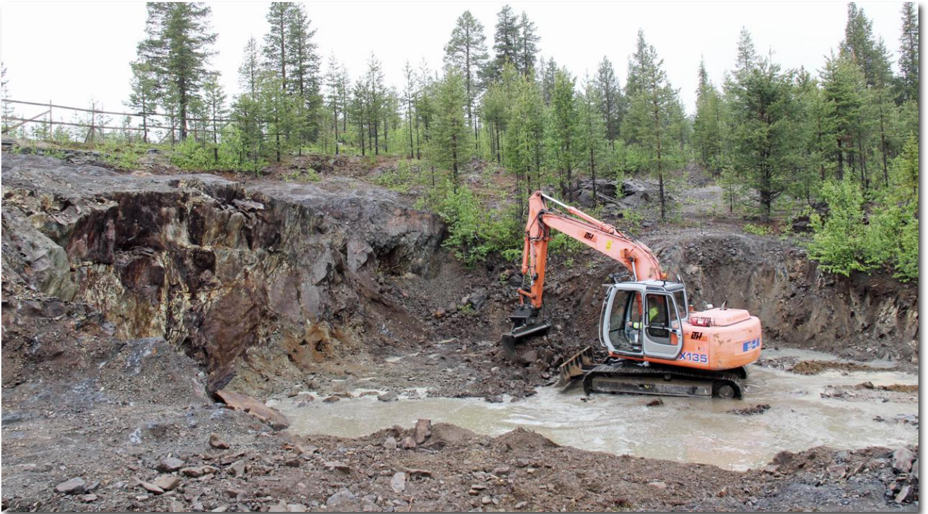
Figure 6 - Site works commence adjacent to historical graphite open cut.
