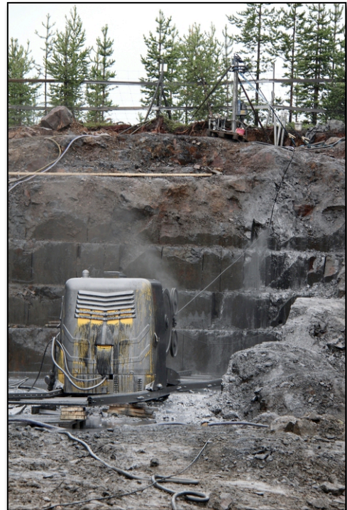
Figure 2 Expanding trial mine benches.
