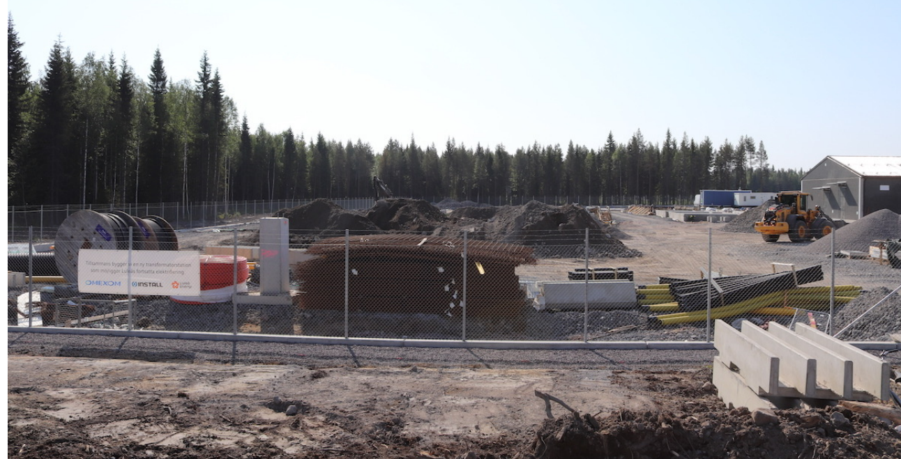
Electrical substation under construction at Luleå Industrial Park
