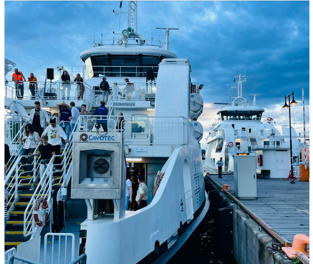
Electric ferry ships in Oslo, 22 August 2022 showing Cavotec battery charger connection.
